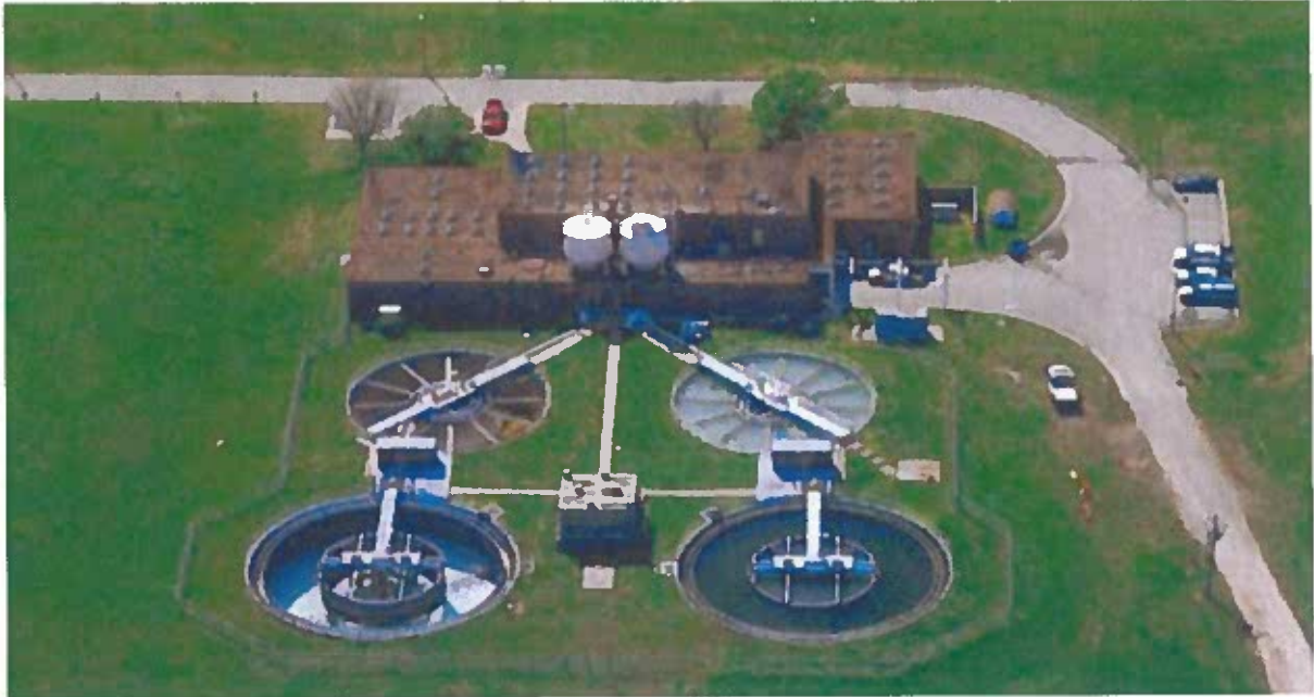
Figure 3.1 Junction City Water Treatment Plant
