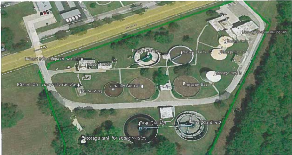
Figure 3.2 East Wastewater Treatment Plant
