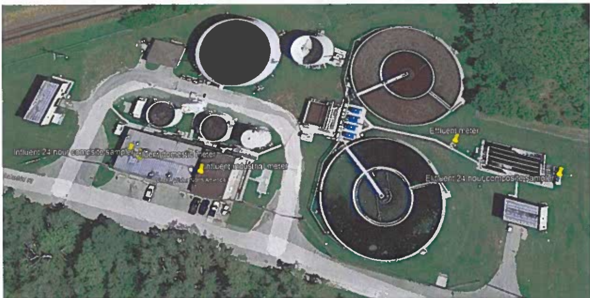
Figure 3.3 Southwest Wastewater Treatment Plant
